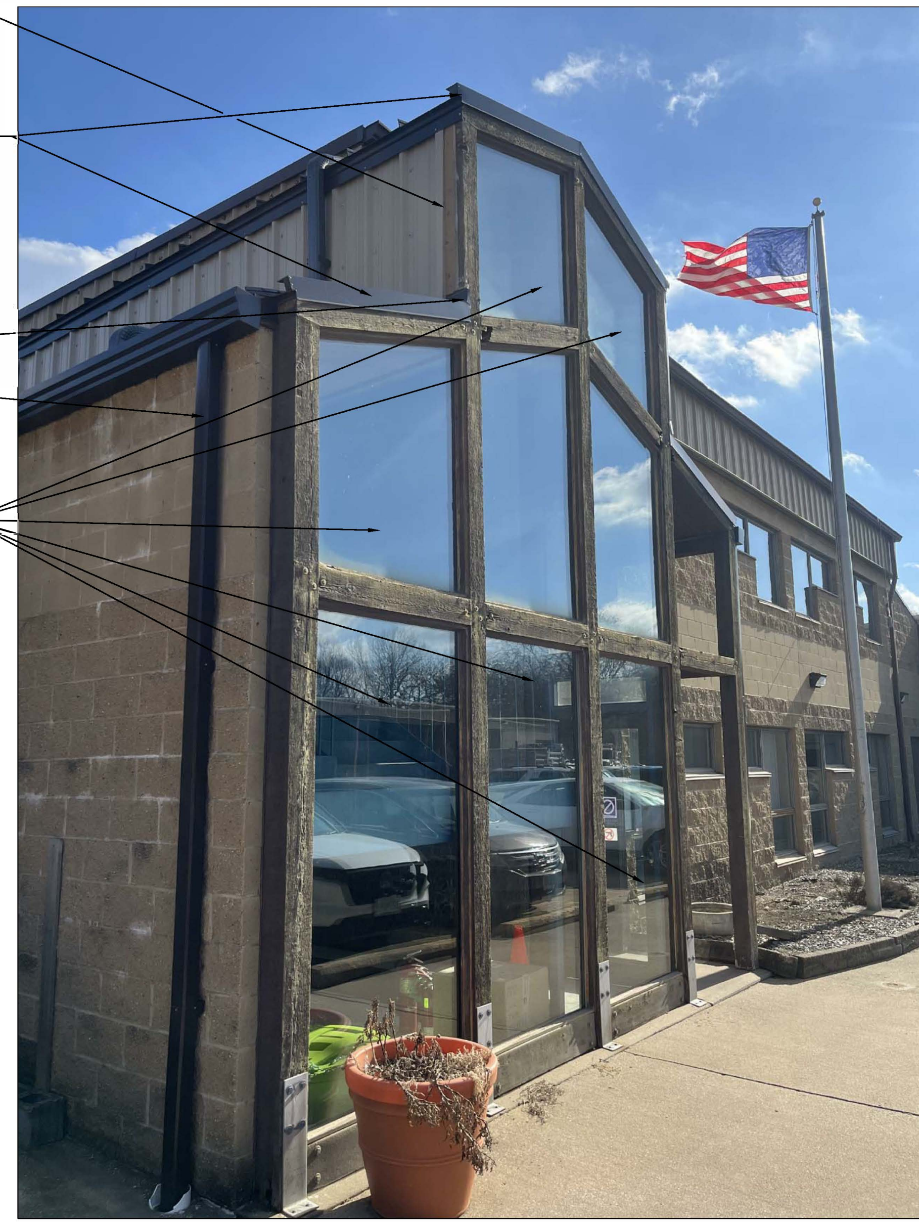
2 EXISTING ENTRY ELEVATION LOOKING SOUTHEAST
