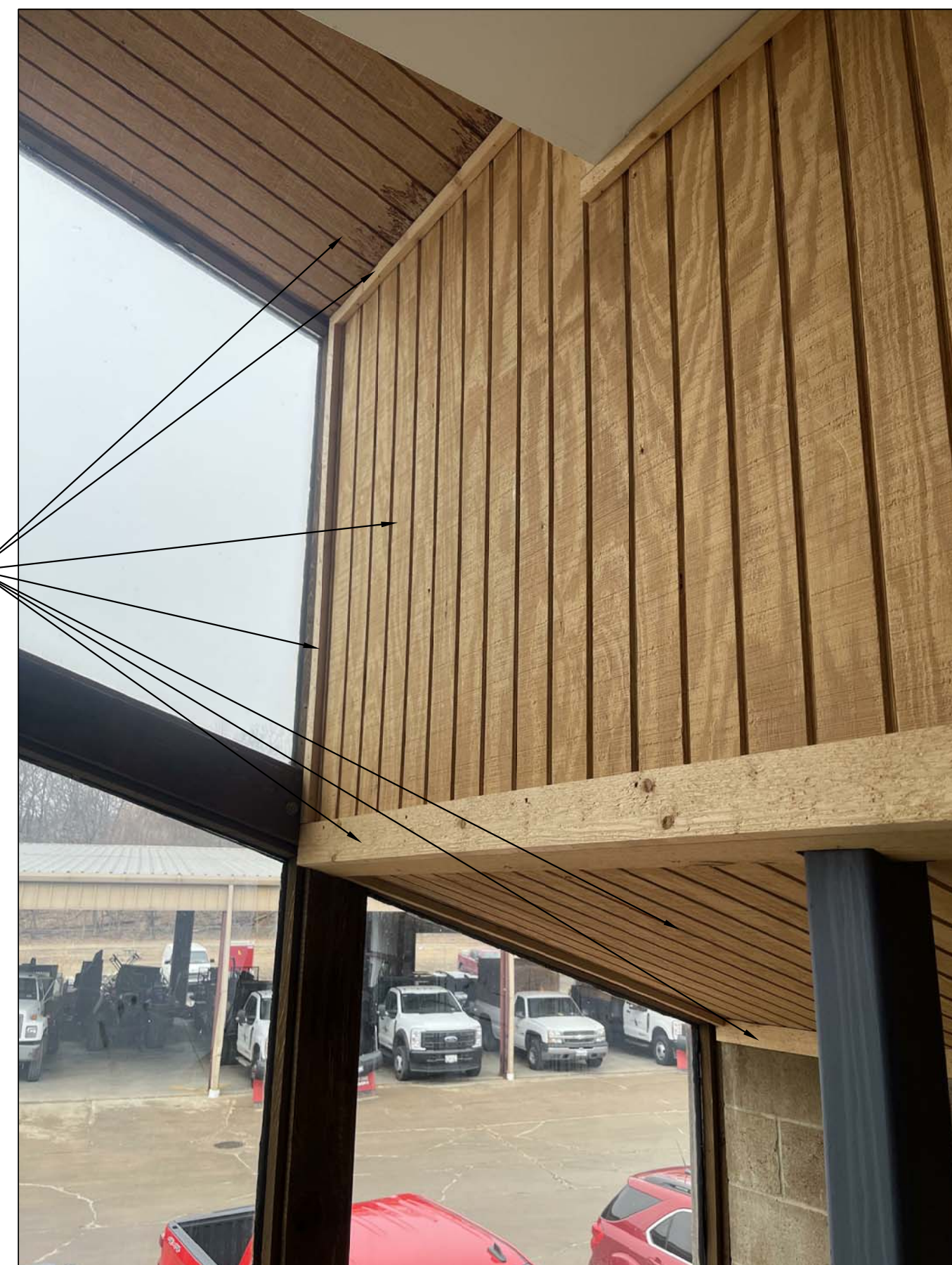
4 EXISTING INTERIOR ELEV. LOOKING NORTHWEST A3 NOT TO SCALE
