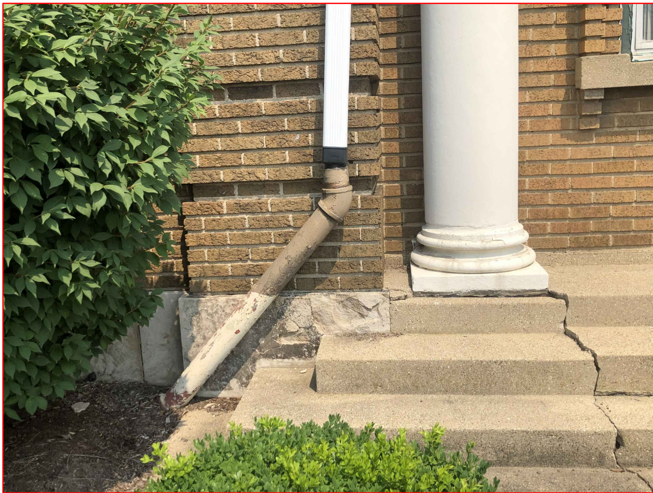
FRONT ELEV. PIC OF STONE FOUNDATION PATCH / REPAIR
