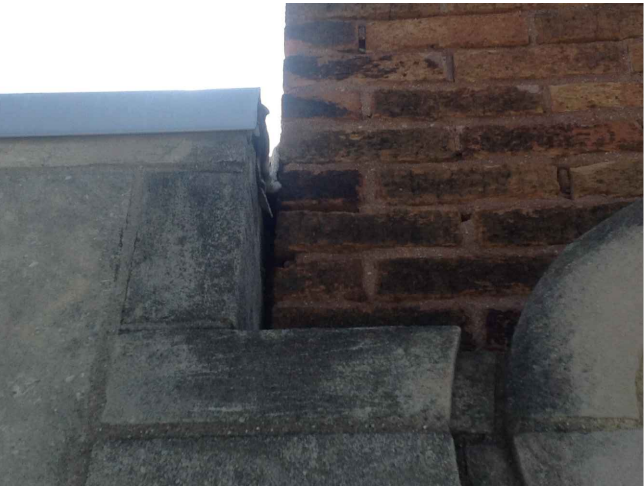
1-10 PARAPET TO BRICK SM. GAP (1 SIM)
