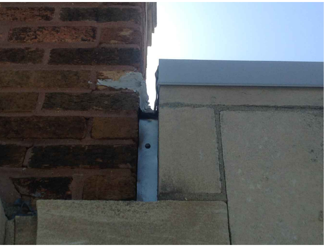
1-11 PARAPET TO BRICK LG. GAP (1 SIM)
